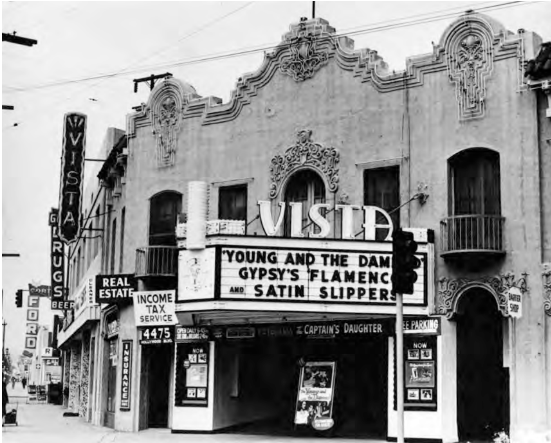
Vista Theatre, 1923 4473 Sunset Boulevard, Los Feliz (Los Angeles Public Library)
